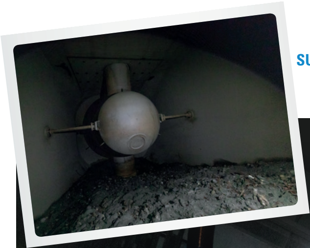
An employee removed around 70 tonnes of gravel and sand in the turbine room
