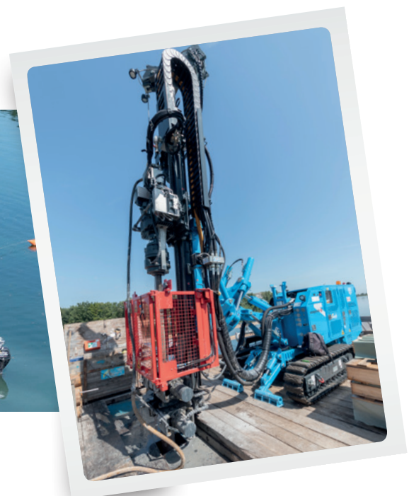
Using a pontoon and drilling device, 20-metre-long drill cores were extracted from the riverbed.
